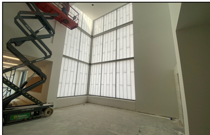
Finishes ongoing in the Chapel.
