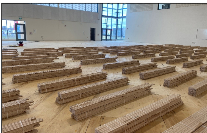
Wood flooring installation in the gymnasium.
